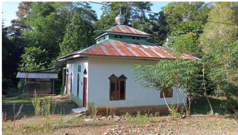
Gambar 2. Masjid Al-Anshar Tampak Belakang
